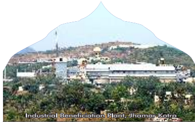
Industrial Beneficiation Plant, Jhama, Kota
