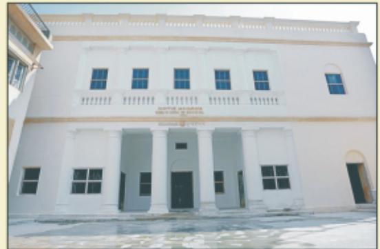
Front facade of the restored Government Girls' Senior Secondary School Jagdish Chowk, Udaipur
