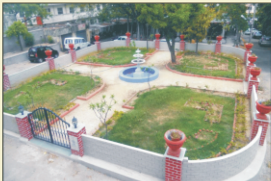
Development of the park at Devasthan Department MG College Road, Udaipur
