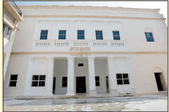
Front facade of the restored Government Girls' Senior Secondary School Jagdish Chowk, Udaipur
